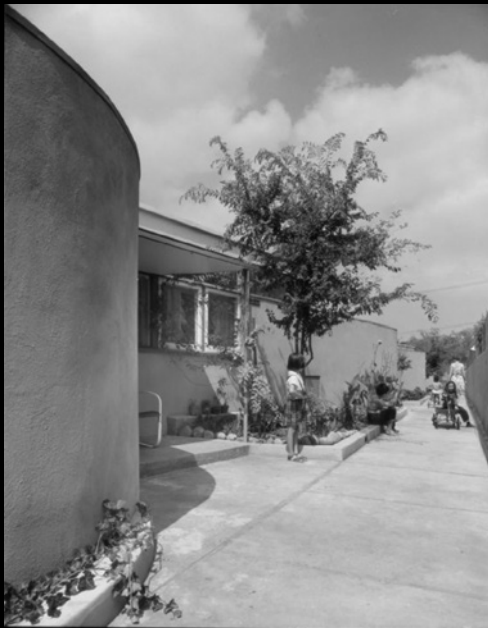
Entry — common walkway looking West at the Avenel Cooperative.
